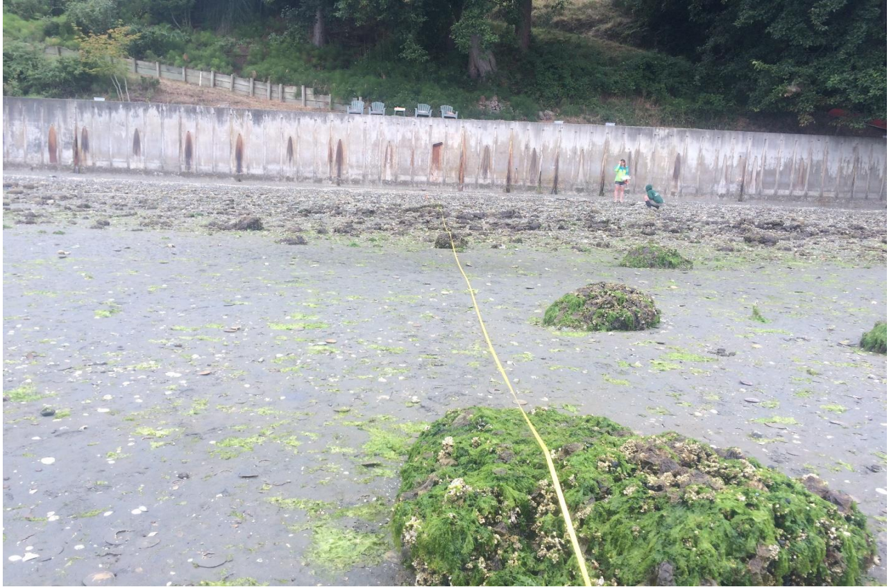
Figure 6 c. Representative photo of the armored treatment at Forest Glen 2016.
